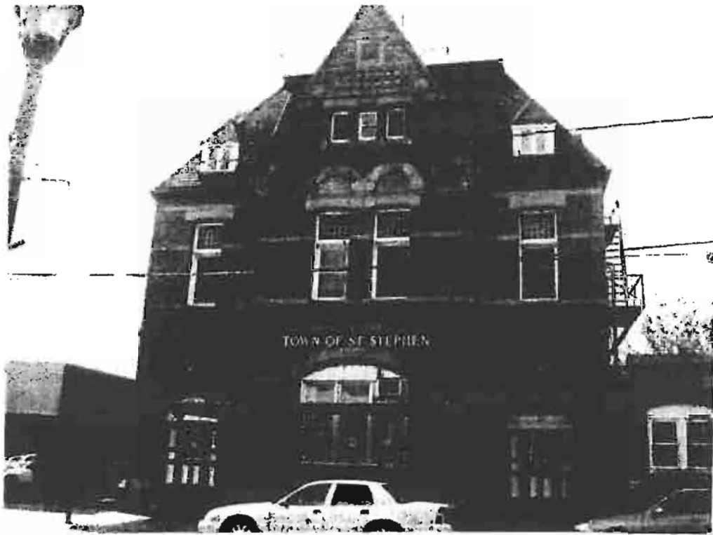
Photo No. 1: North, (Front), Elevation of Building. (2014-05-23)
