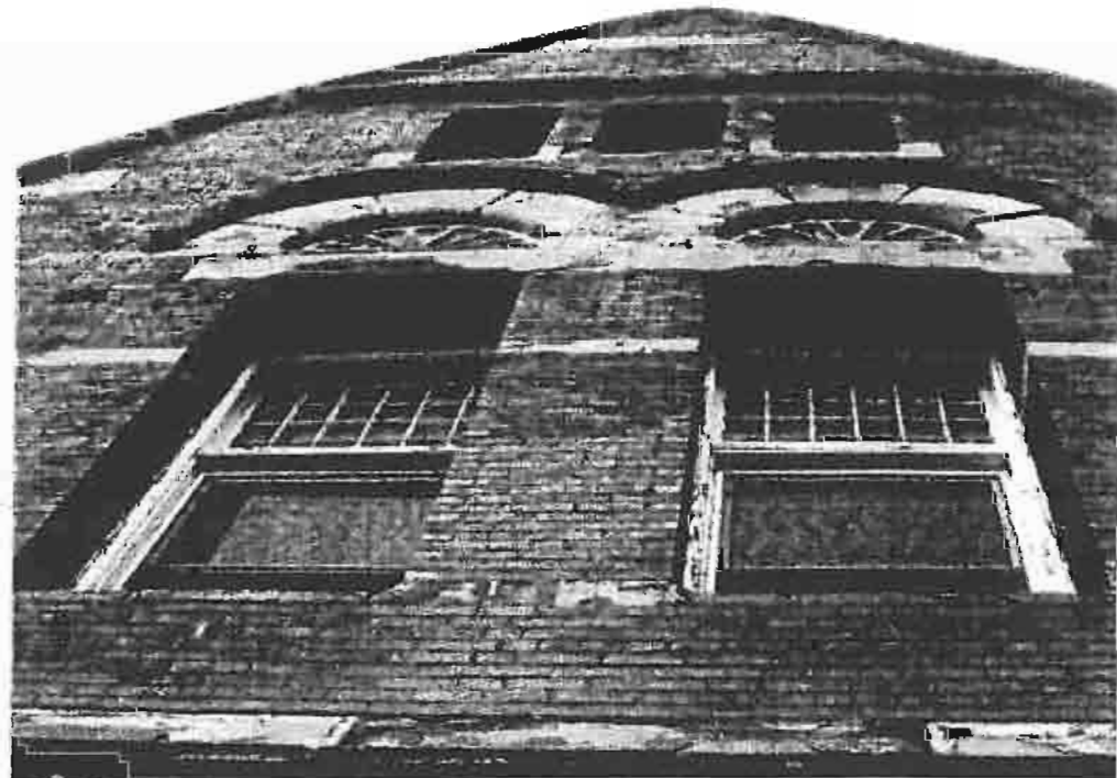
Photo No. 8: East Elevation of Building. (2014-05-23)
